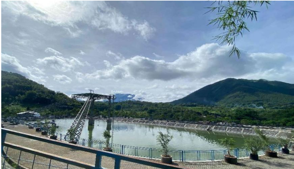
Figure 6.23 Application of Water Reservoir
