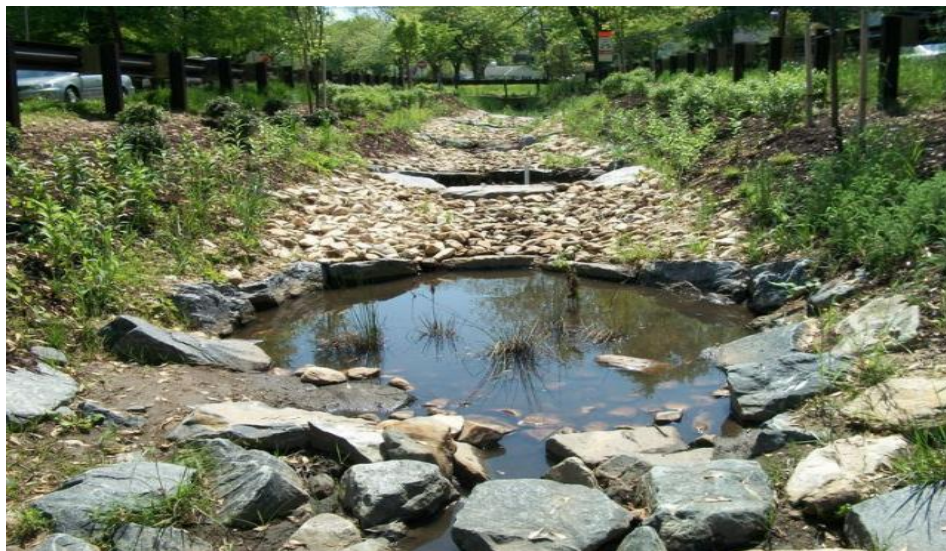
Figure 6.10 Loose Stone Check Dam
