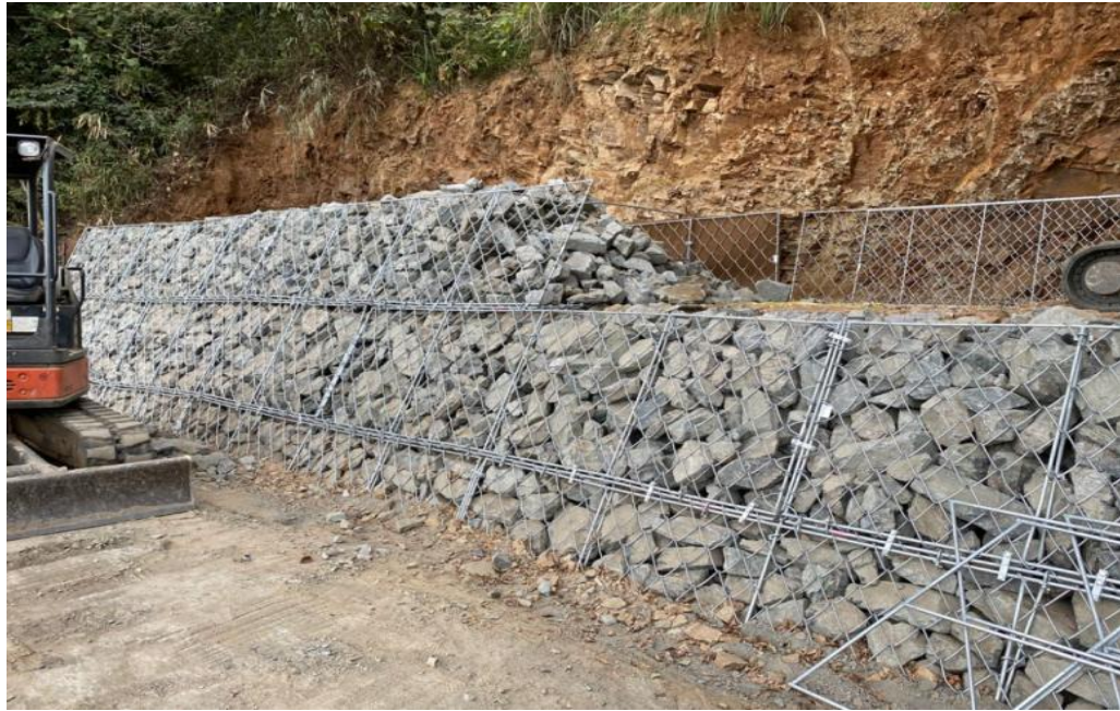
Figure 6.11 Gabion Check Dam
